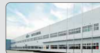
Fujitsu General Central Air Conditioner (Wuxi) Co. Ltd.
