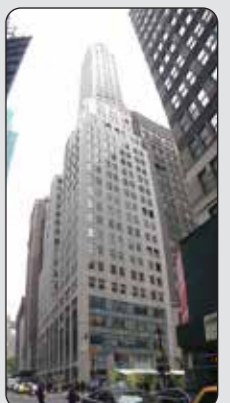
Fujitsu General Solution Centre "THE AIRSTAGE"
