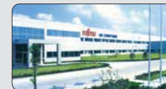
Fujitsu General (Shanghai) Co. Ltd.
